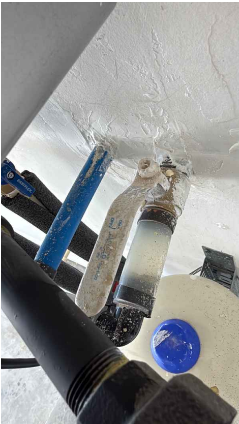
A. Plumbing Supply, Distribution Systems, and Fixtures: Type of Supply Piping Material PEX
