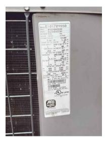
Approximate Condensing Unit BTU/Tonnage: 4 TON
