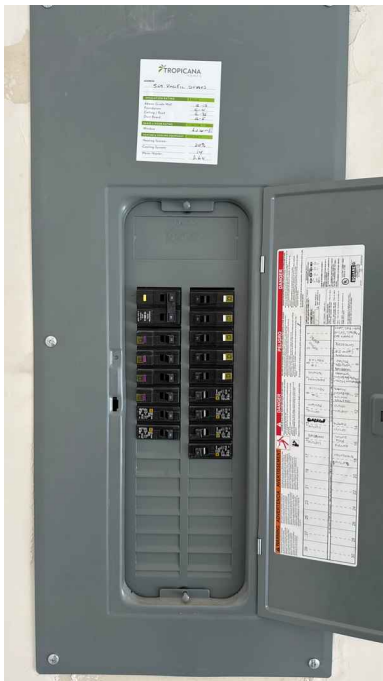
Sub-Panel Location: Garage Sub-Panel Amperage: 100 Amp Sub-Panel Manufacturer: Square D
